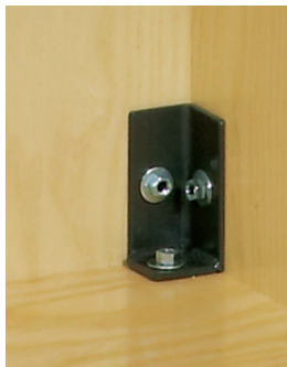
Two, triple-bolted corners for extra strength
